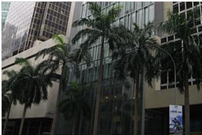
135 Cecil Street: Pricing said to be around $2,200 psf on existing net lettable area. - FILE PHOTO
